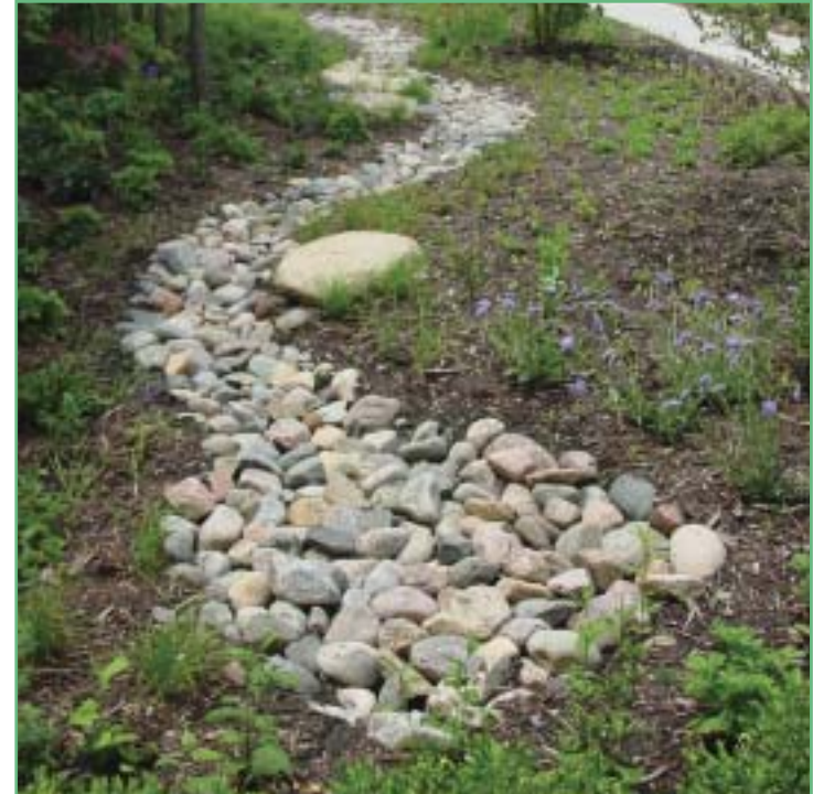
Drainage swales are one of the Best Management Practices that can effectively move water from parking and other areas.
