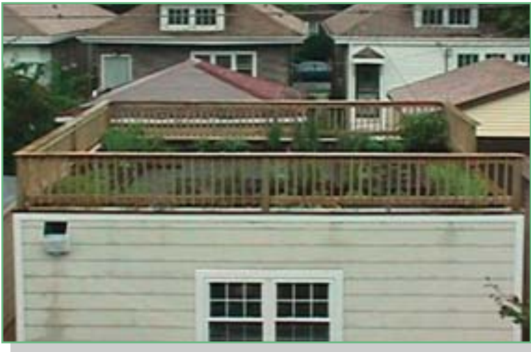
Chicago's Green Bungalows program encourages the use of green roofs. Green roofs are one of the many BMPs that will be recommended in this guide to handle stormwater runoff.
